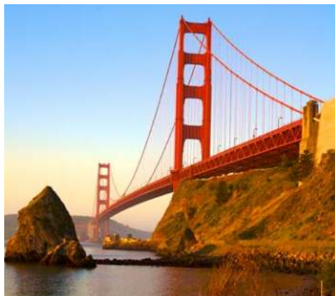
Golden Gate Bridge
